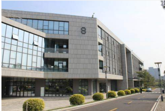
Songshan Lake Office Building
